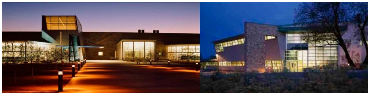
Figure 2.1 CINT Core Facility (left) and Gateway Facility (right).
