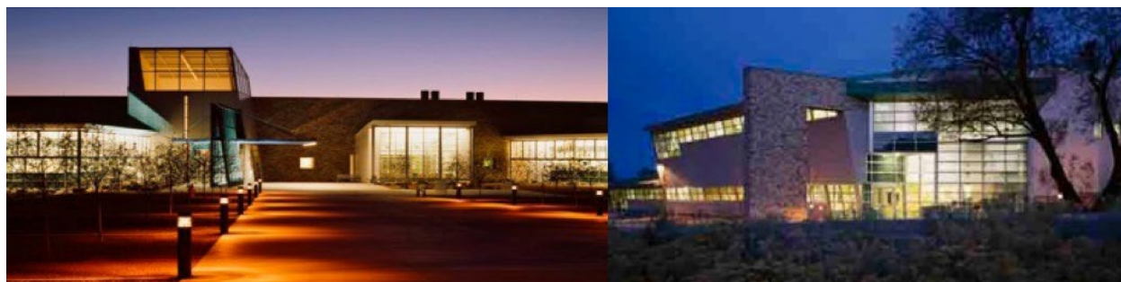
Figure 2.1 CINT Core Facility (left) and Gateway Facility (right).
